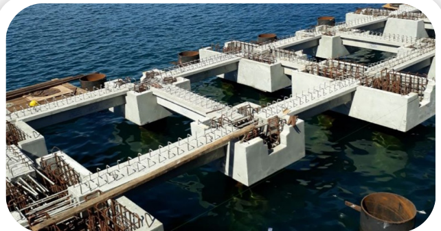
● Jetty Construction Piabung Port
