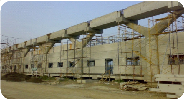
● Beam Column Slab System (BCS) Sampoerna Warehouse Karawang
