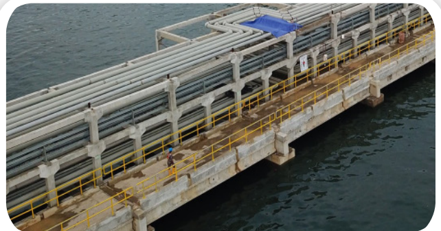
● Pipe Rack Tanjung Batu Balikpapan Jetty
