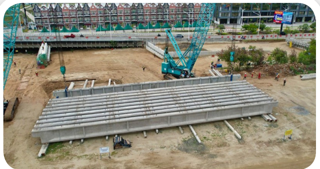
● PCI Girder C-D Island Connection Bridge Pantai Indah Kapuk 2
