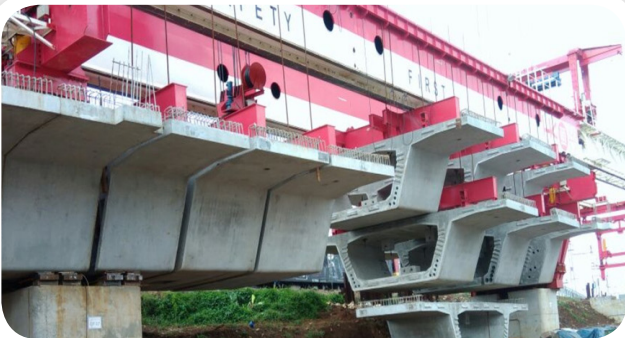
● Box Girder Double Double Track Manggarai
