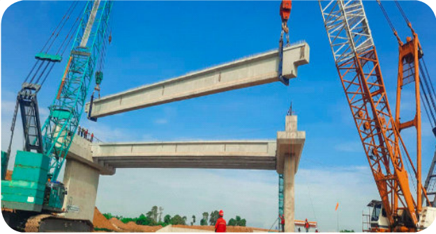
● PCI Girder Probolinggo Banyuwangi Toll Road
