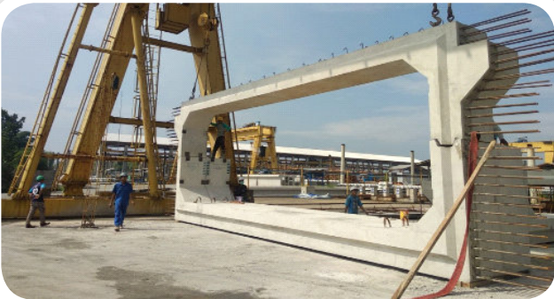
● Box Culvert Grenyang Bojonegoro Bridge
