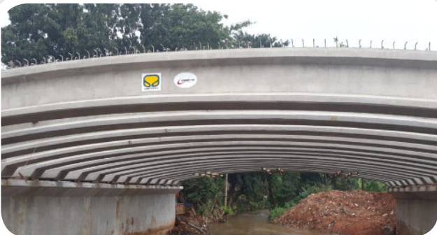
● Curved PCI Girder UIII Campus Main Gate Bridge Depok
