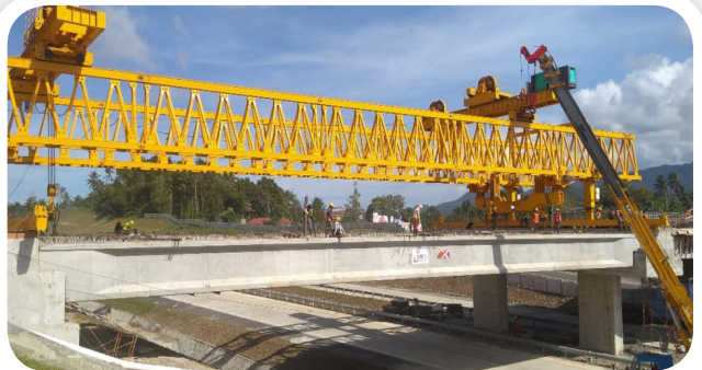
● PCI Girder Manado Bitung Toll Road
