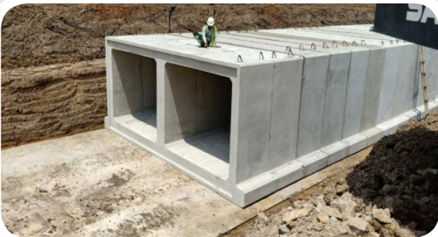
● Box Culvert New Yogyakarta International Airport
