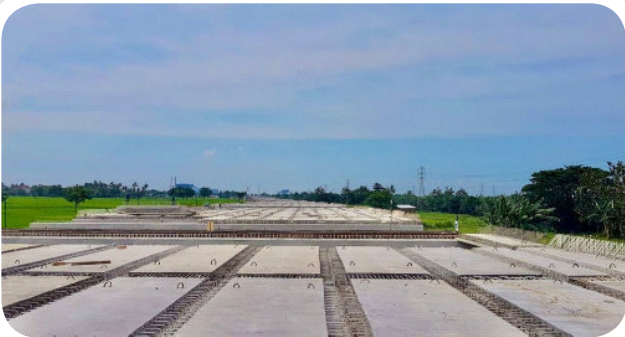
● Full Slab Cibitung Cilincing Toll
