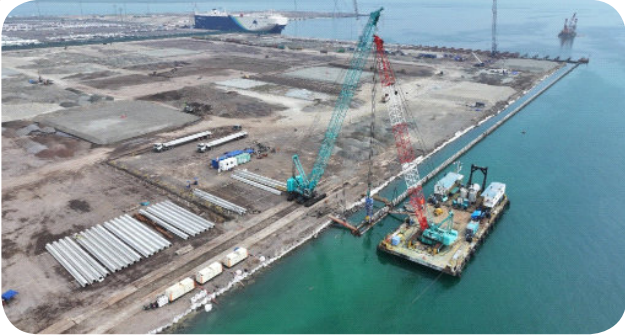
● Corrugated Concrete Sheet Pile (CCSP) Patimban Port
