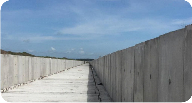
● U-Ditch Yogyakarta Airport
