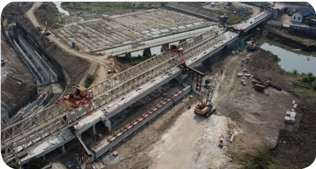
● PCI Girder Glapan Timur Rehabilitation
