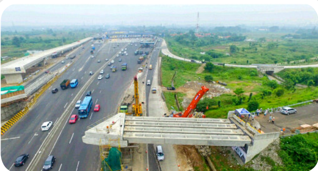
● PCU Girder Over Pass Dry Port Cikarang
