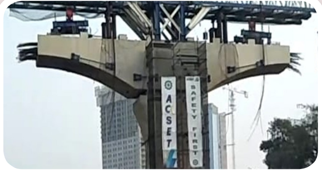
● Pier Head Precast Jakarta - Cikampek 2 Elevated Toll Road
