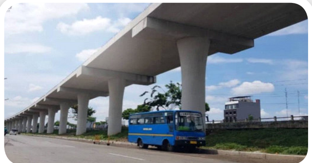
● Voided Slab JLNT Pluit By Pass
