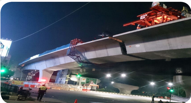
● Box Girder Pancoran Fly Over
