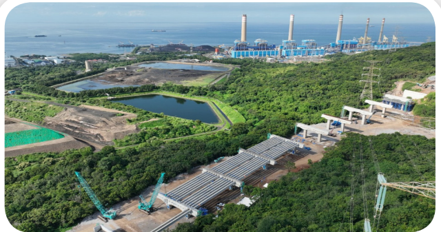
● PCI Girder Probolinggo Banyuwangi Toll Road
