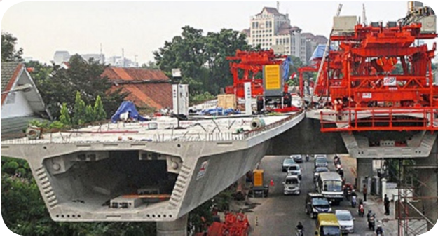
● Box Girder Bogor Outer Ring Road
