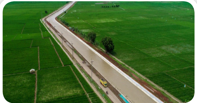
● Lining Anjatan Sukro Irrigation
