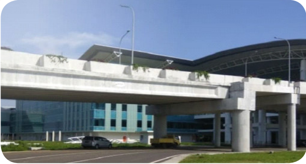
● Voided Slab Entrance Access Kertajati Airport
